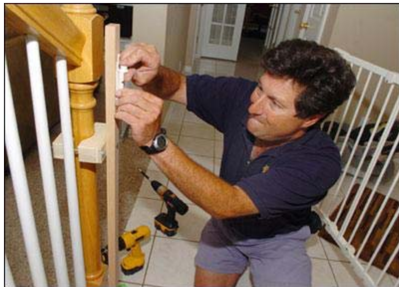
Lou Delaware, owner of Colorado Childproofers, installs a staircase gate in a house in Lafayette, using techniques that don't damage the rails and posts. (Post / John Epperson)
